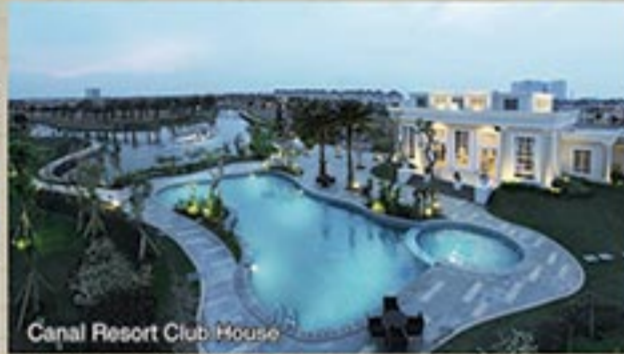
Canal Resort Club House
